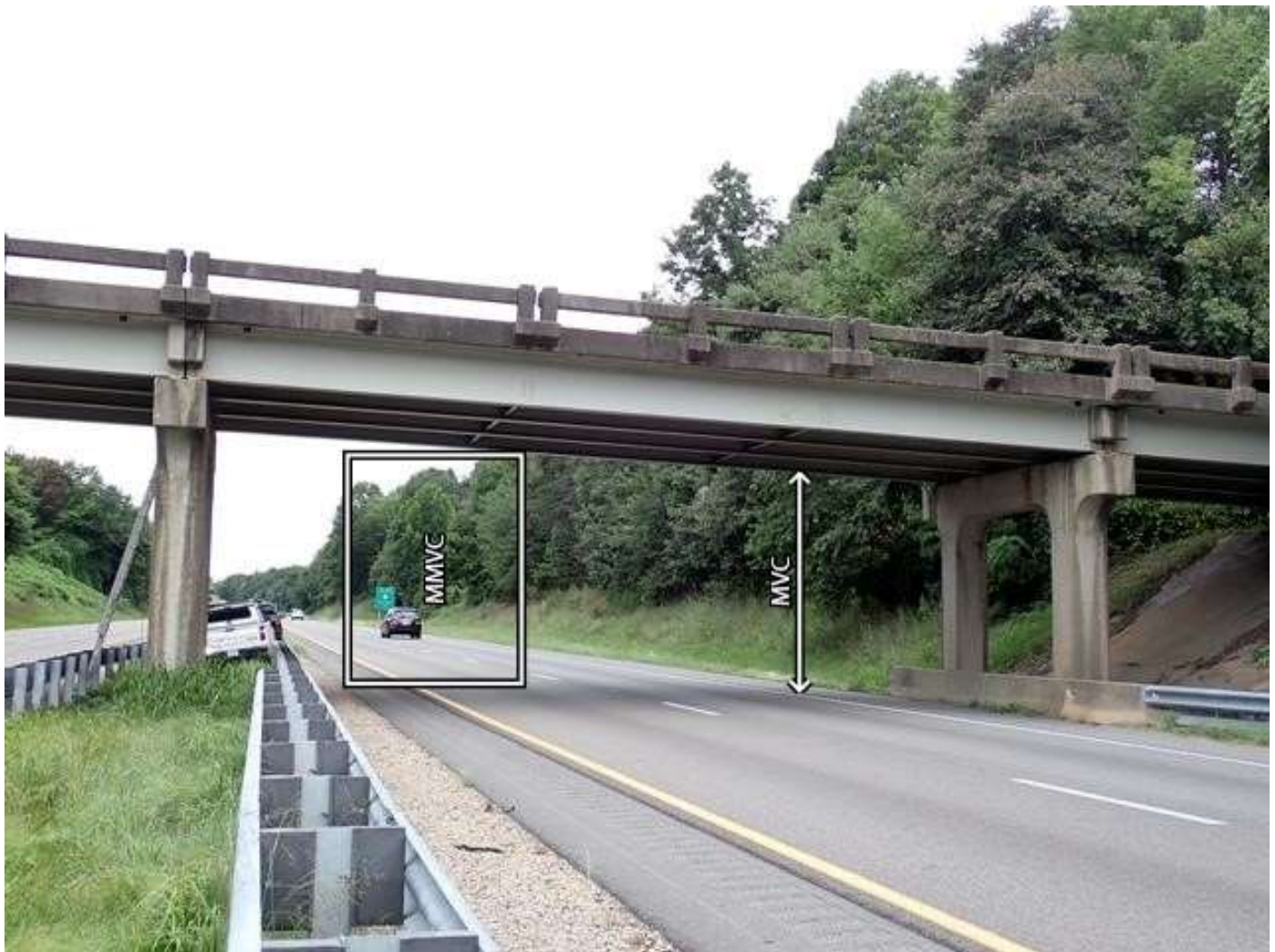
roadway under span 3, looking west (I-40 westbound)
