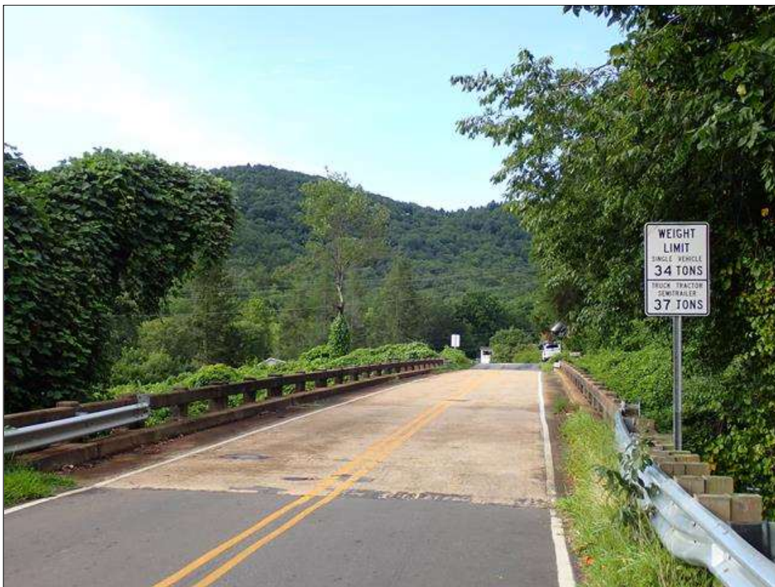
north approach looking south
