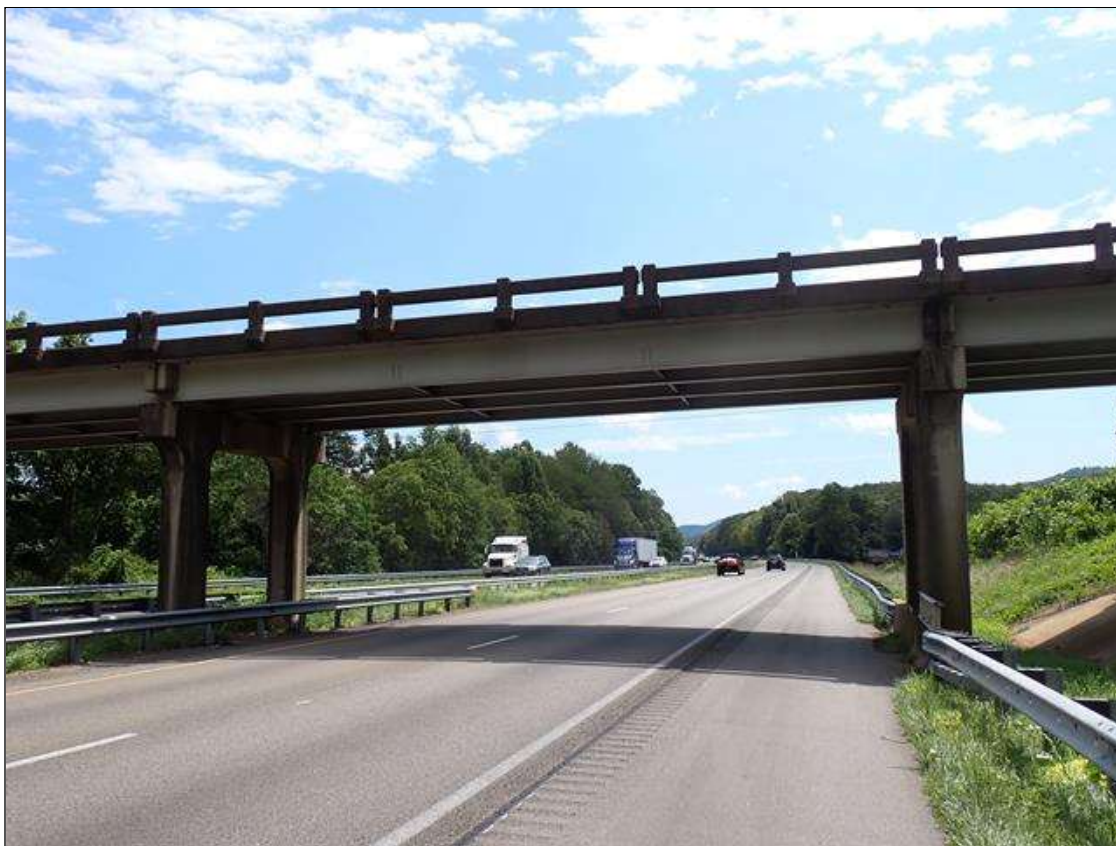
roadway under span 2, looking east (I-40 eastbound)
