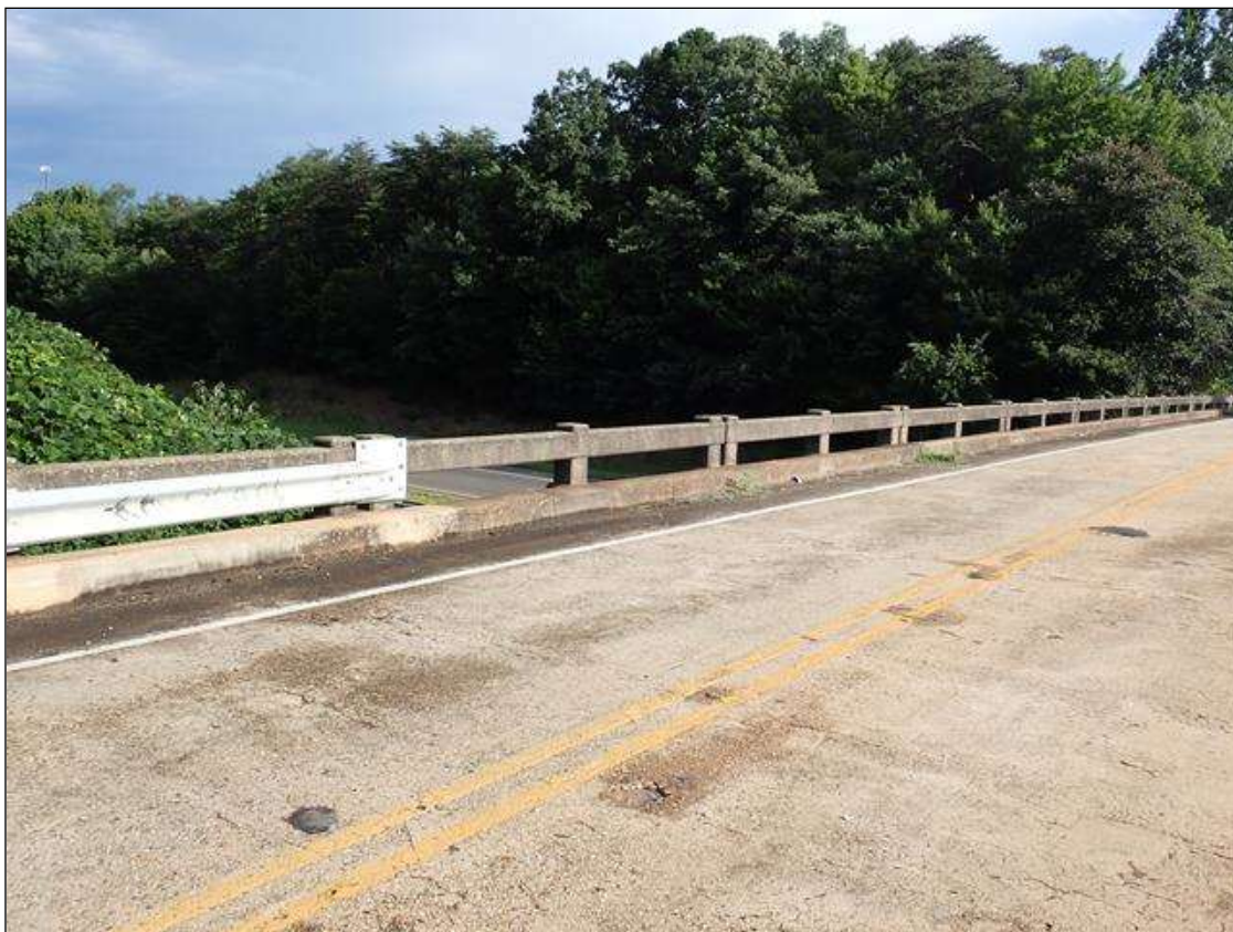
left bridge rail
