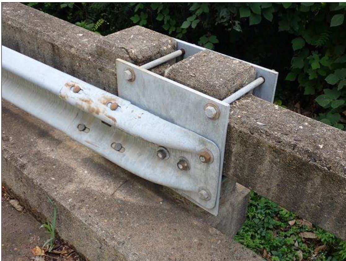
northeast guardrail attachment
