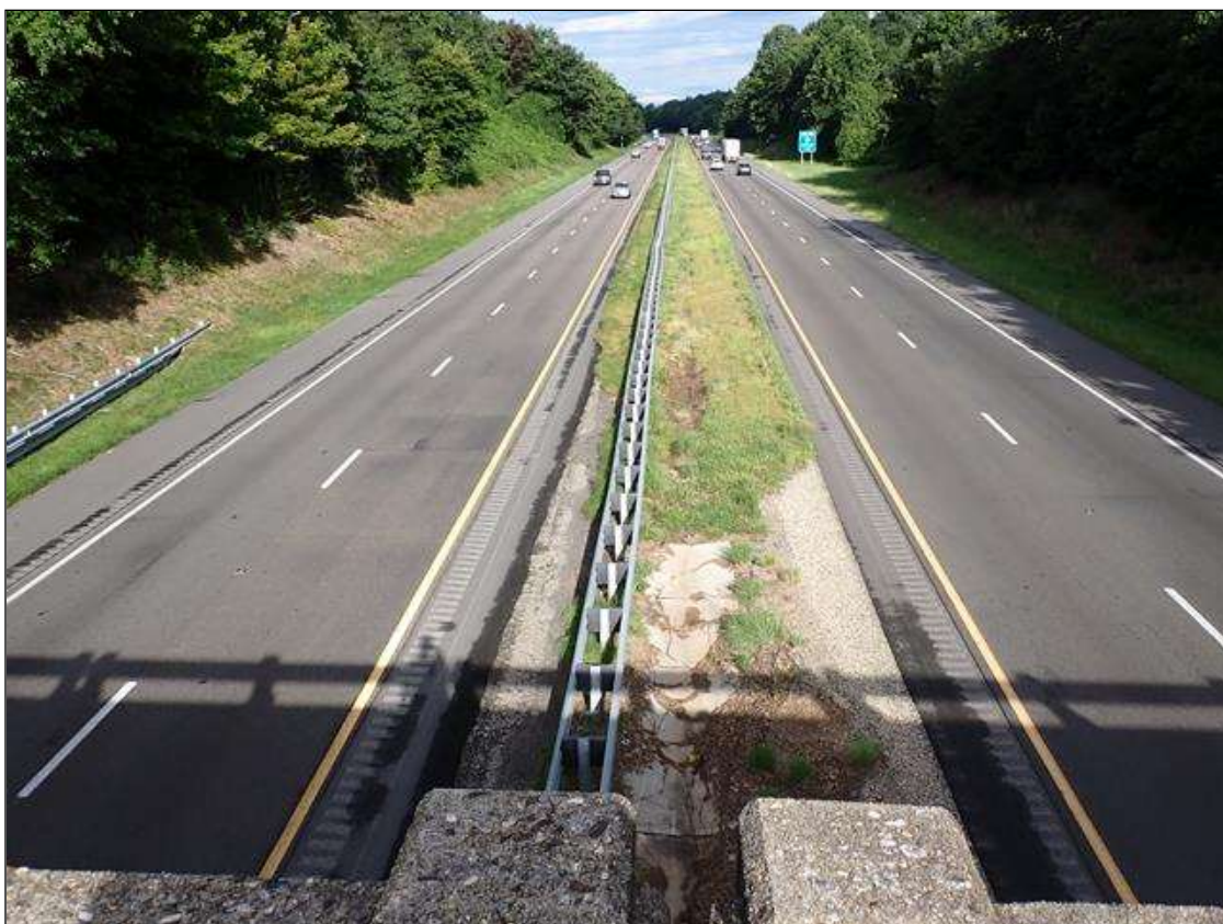
roadway looking west
