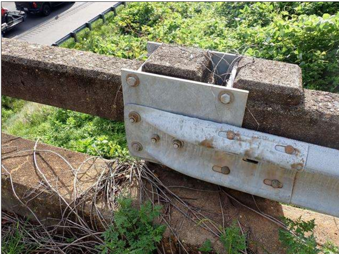
southeast guardrail attachment
