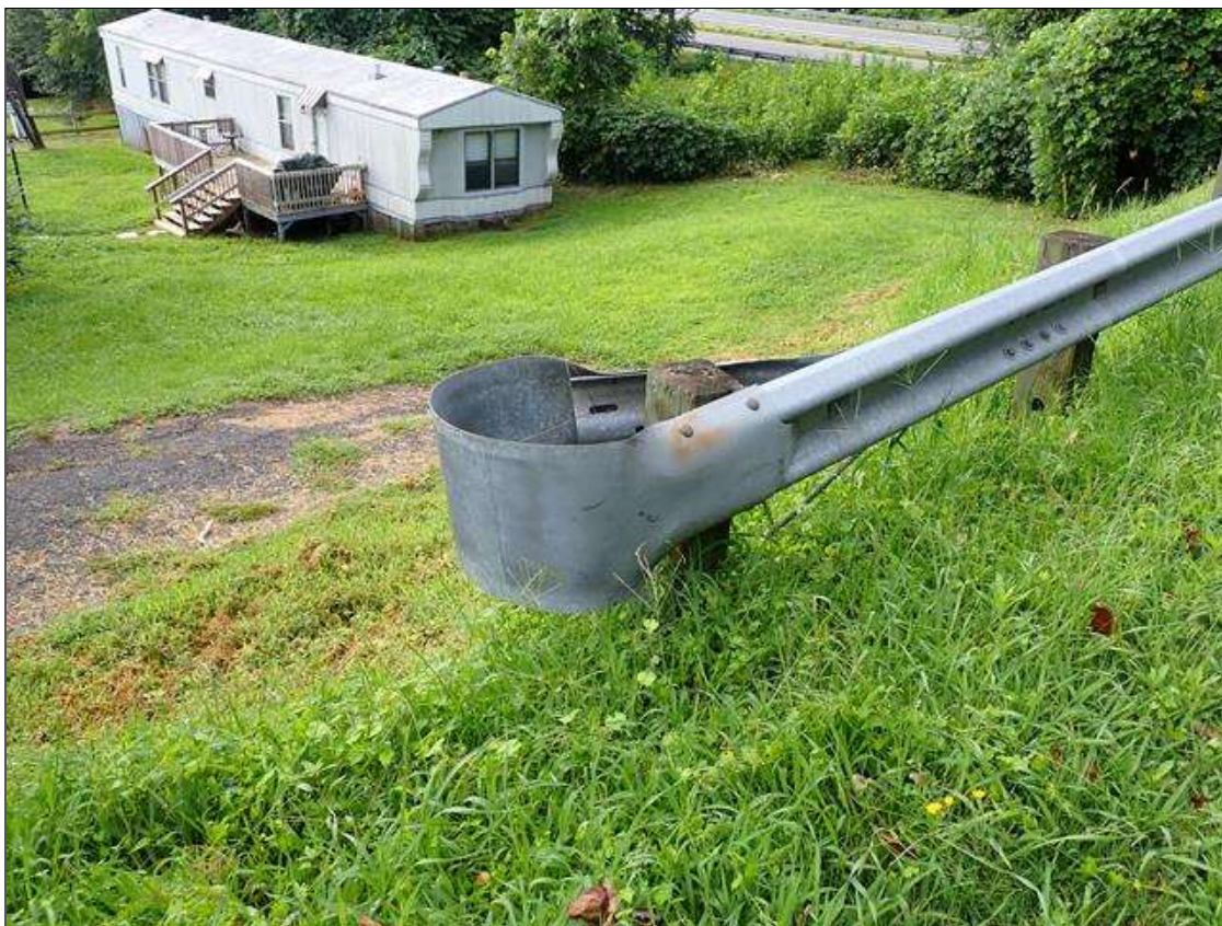
northeast guardrail termination
