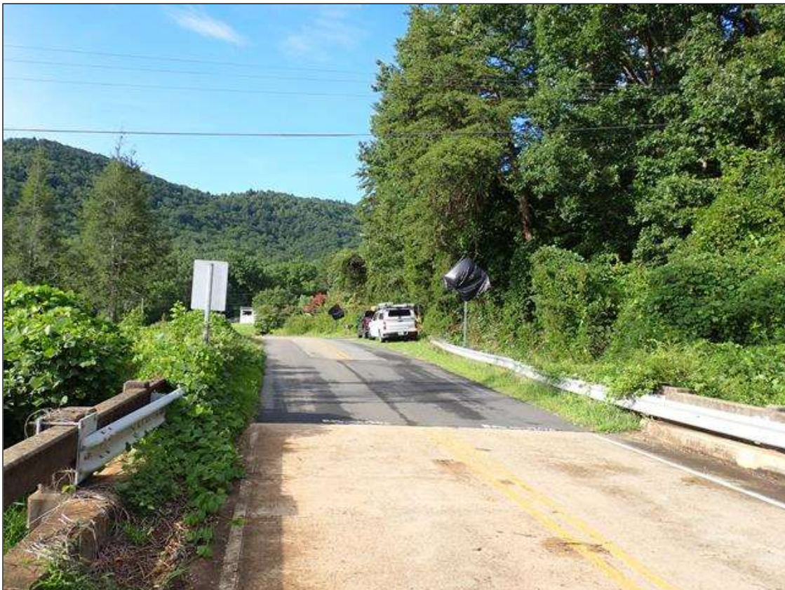
south approach looking south
