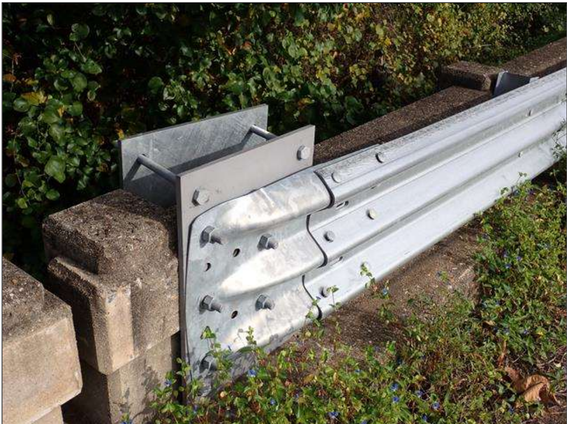
northwest guardrail attachment
