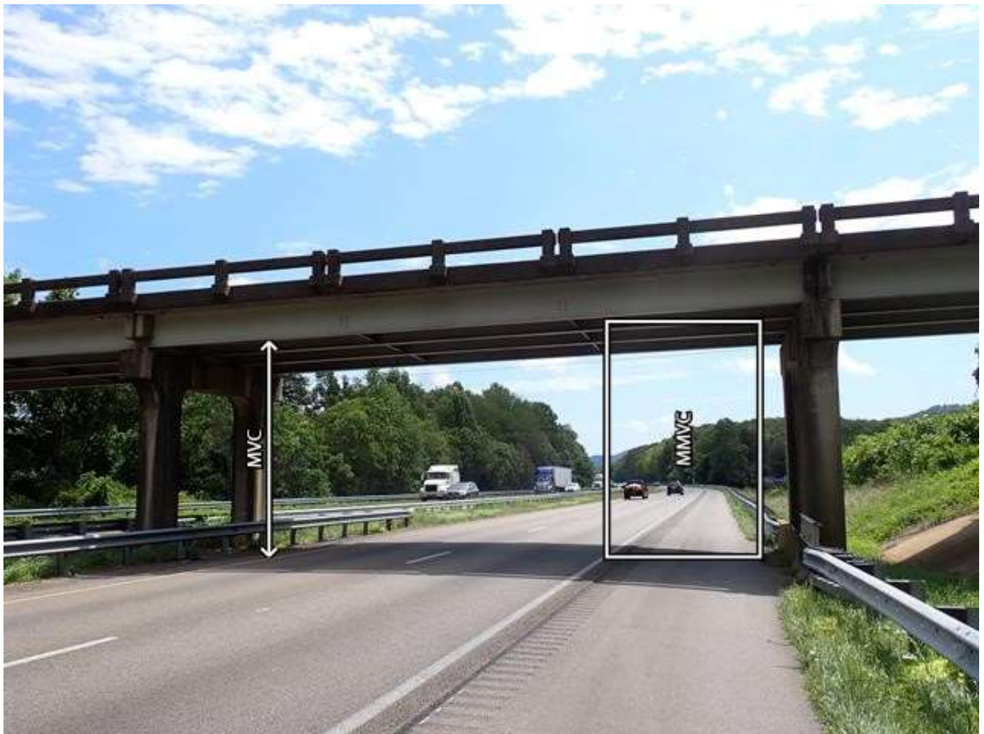
roadway under span 2, looking east (I-40 eastbound)
