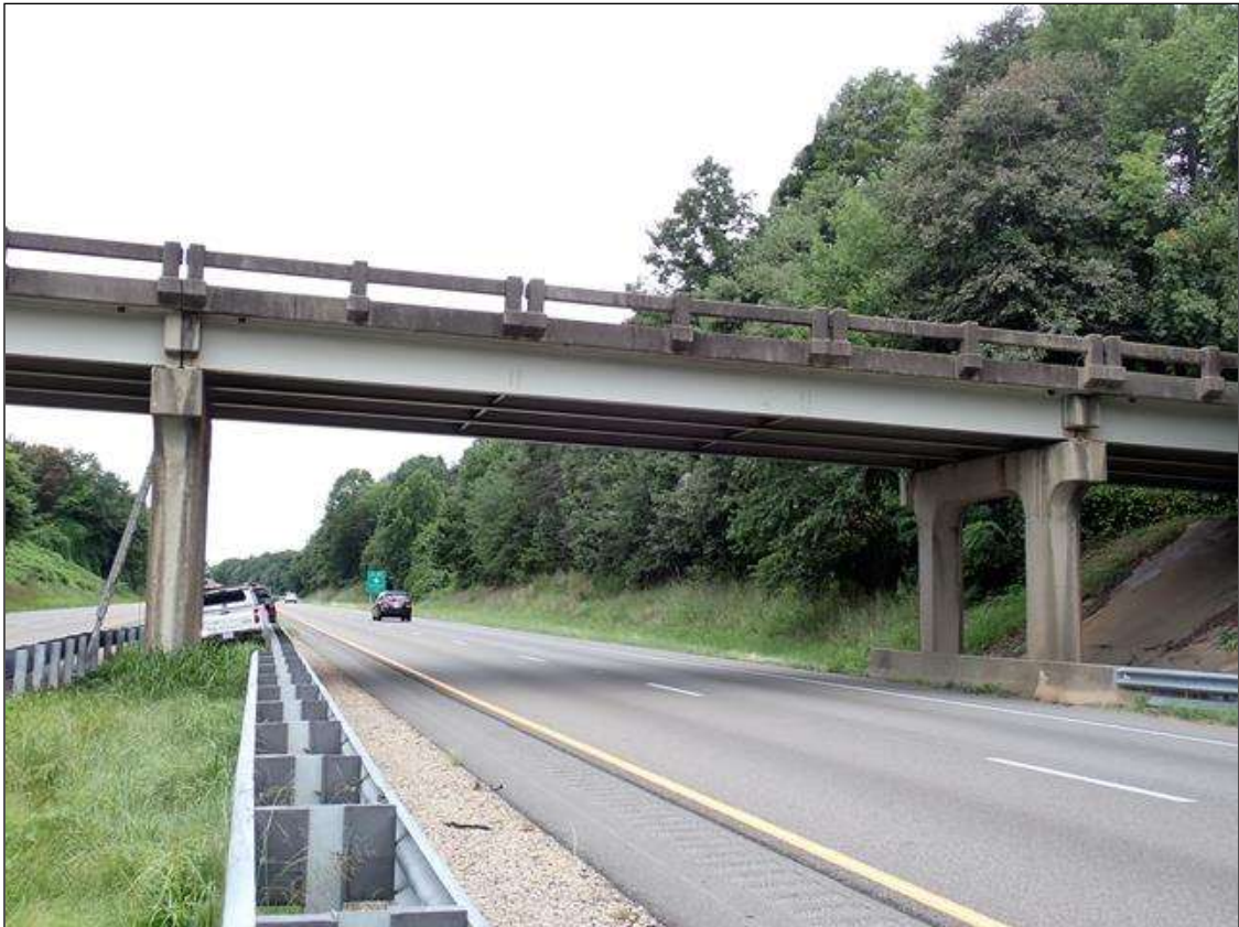
roadway under span 3, looking west (I-40 westbound)
