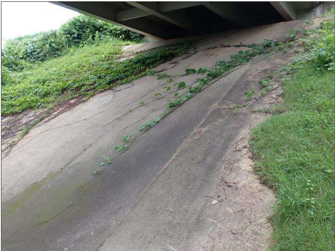
end bent 1 slope protection
