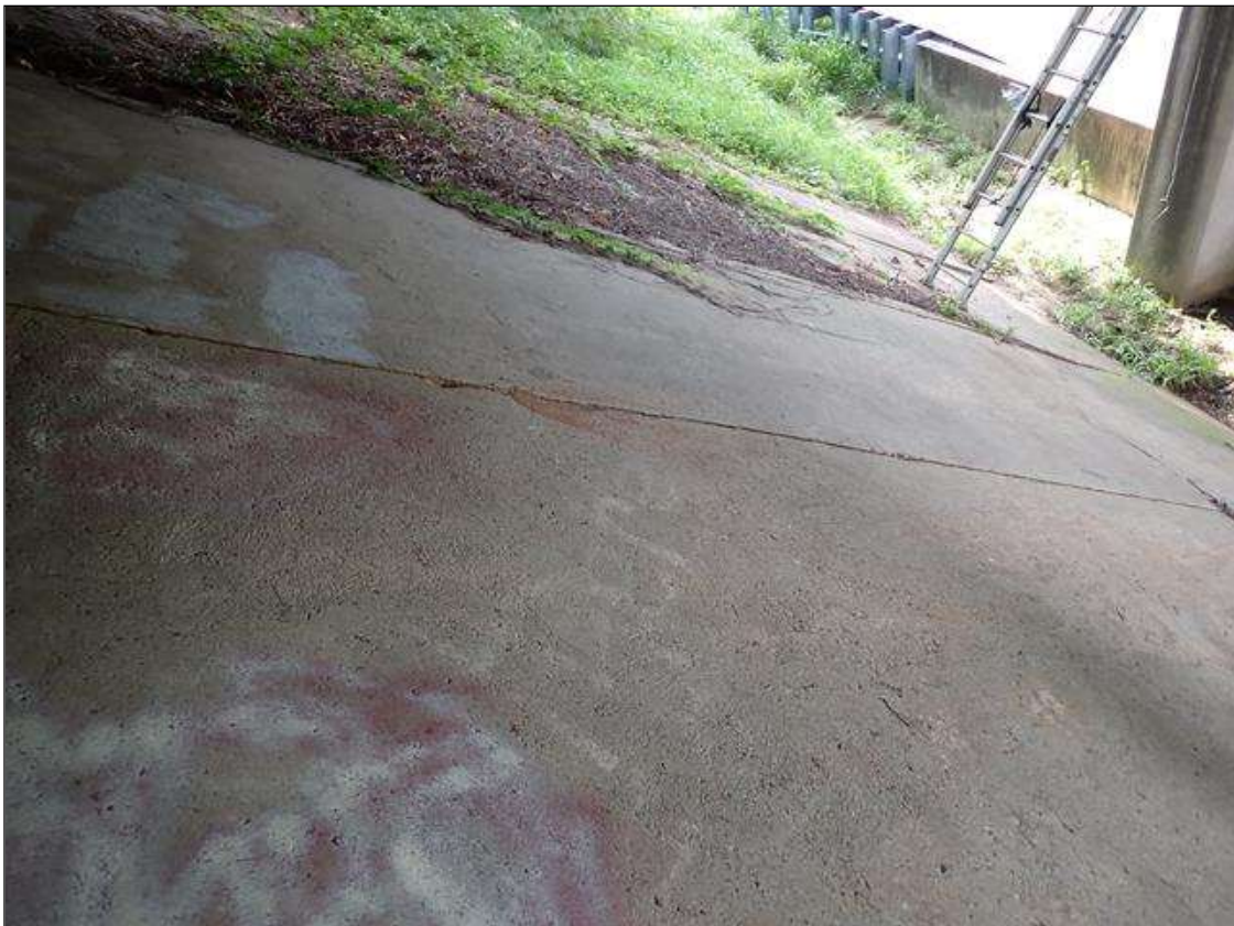
end bent 2 slope protection
