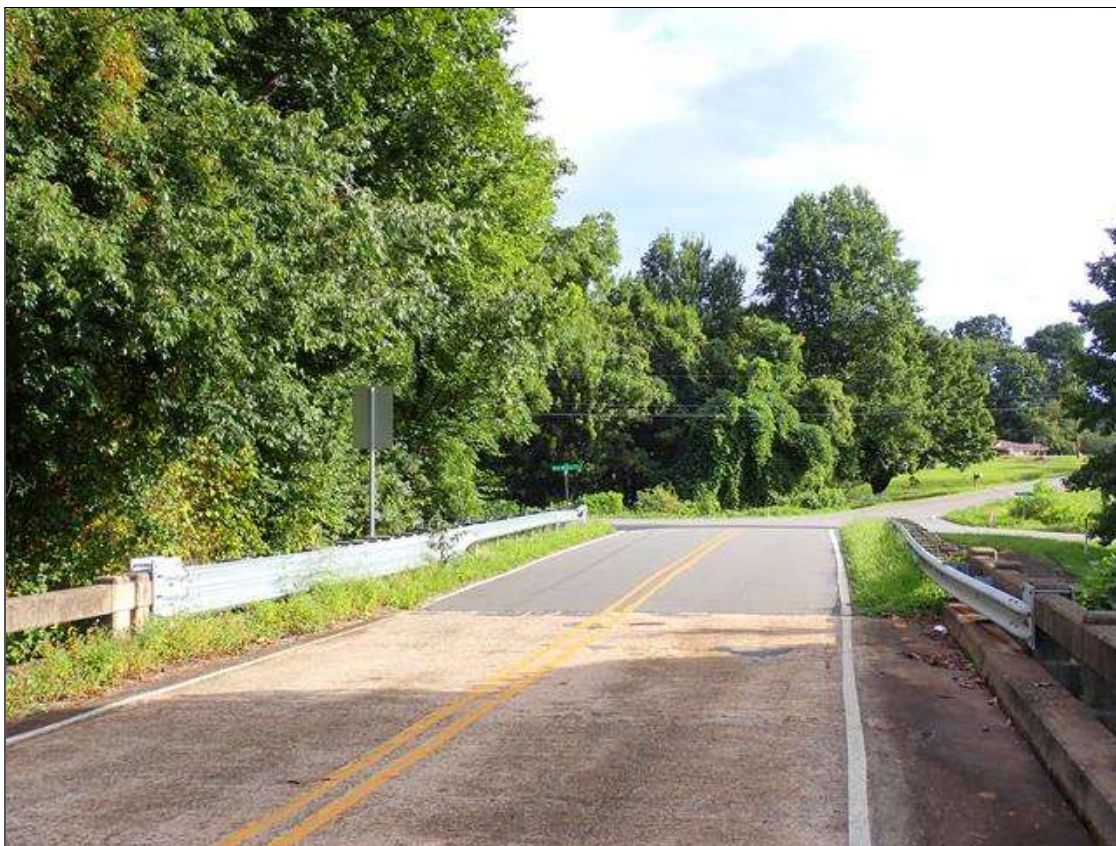
north approach looking north
