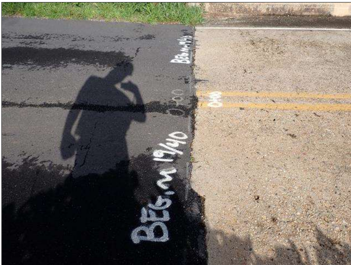
end bent 1 deck
