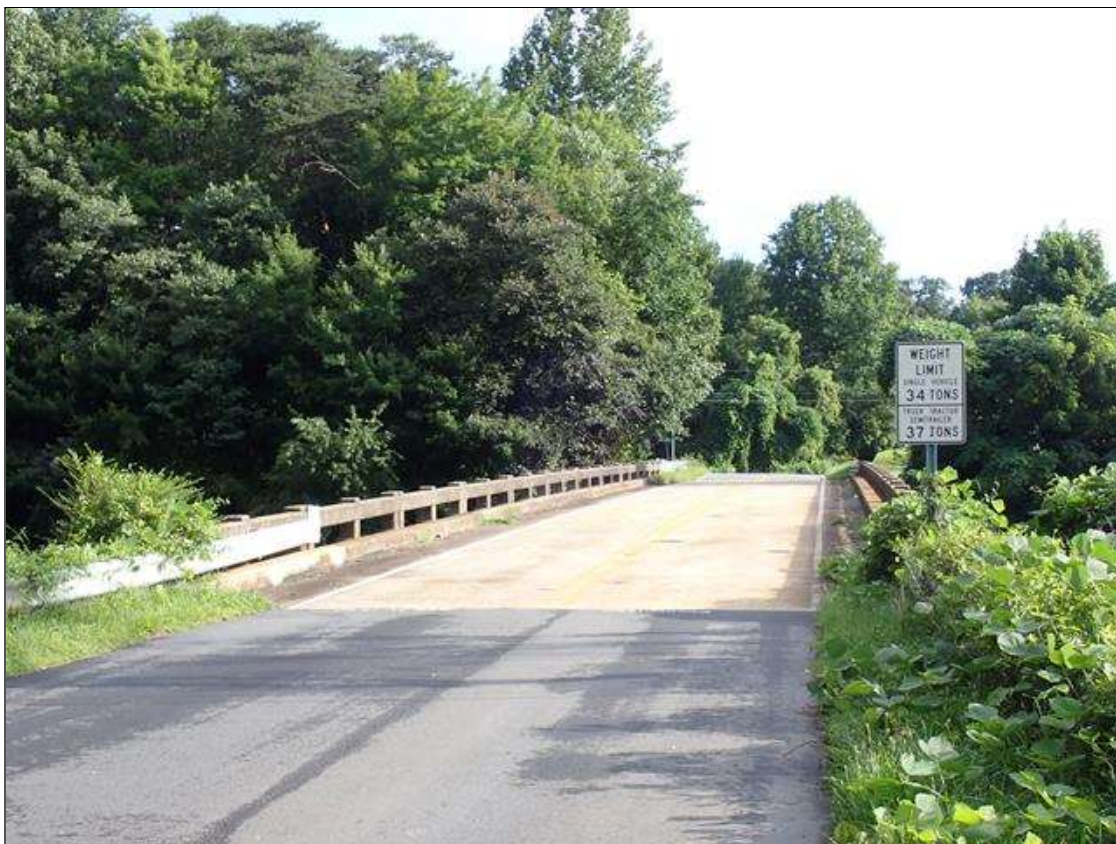
south approach looking north
