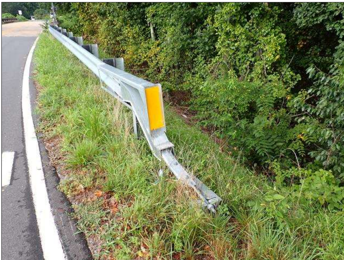
northwest guardrail termination
