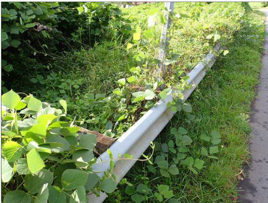
southeast guardrail transition
