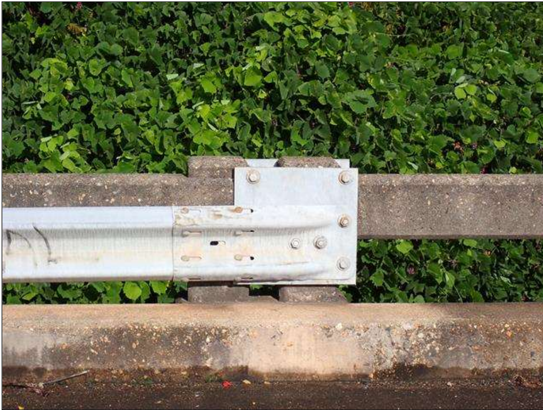
southwest guardrail attachment
