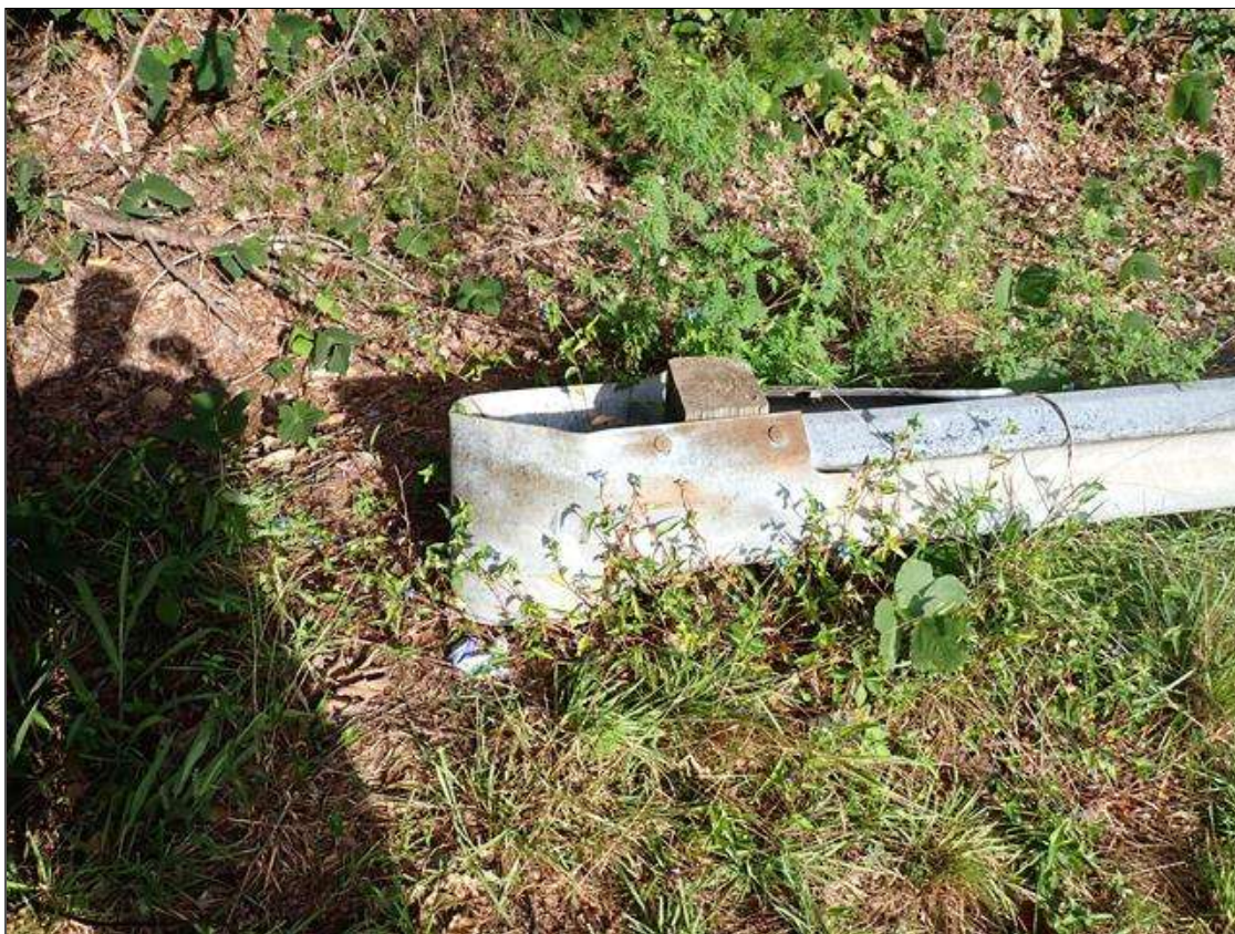
southwest guardrail termination
